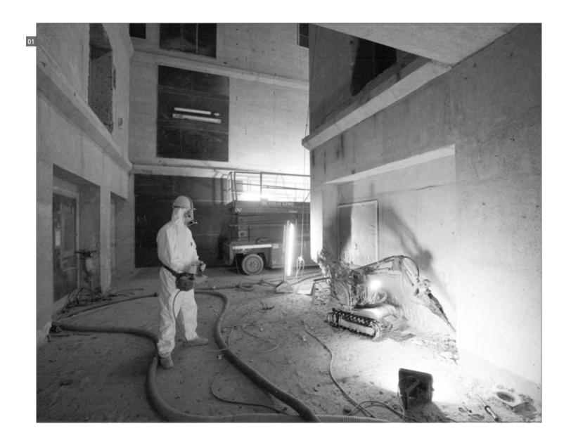
Remote controlled demolition hammers are used to remove subsurface contamination in walls and floors.
