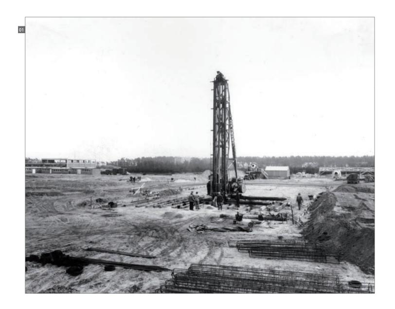
Sinking the foundation piles. To prevent water from seeping in the installations during flooding, the ground level was raised.
